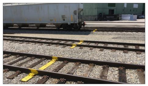
2. *MRH* forum member **Ken Rice** started a thread about how the prototype marks track clearance points. He posted this photo and is encouraging others to post more photos to show different methods used by real railroads for this.
