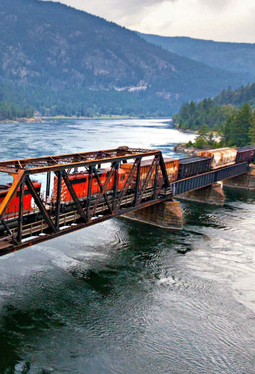
A westbound Canadian Pacific freight from Nelson bound for the smelter at Trail, B.C., crosses the Kootenay River at Taghum. This bridge, which inspired a model on Mark Dance's N scale Columbia & Western Ry., comprises nine spans of varying styles and crosses two islands over a distance of 763 feet. Matthew Hicks photo
