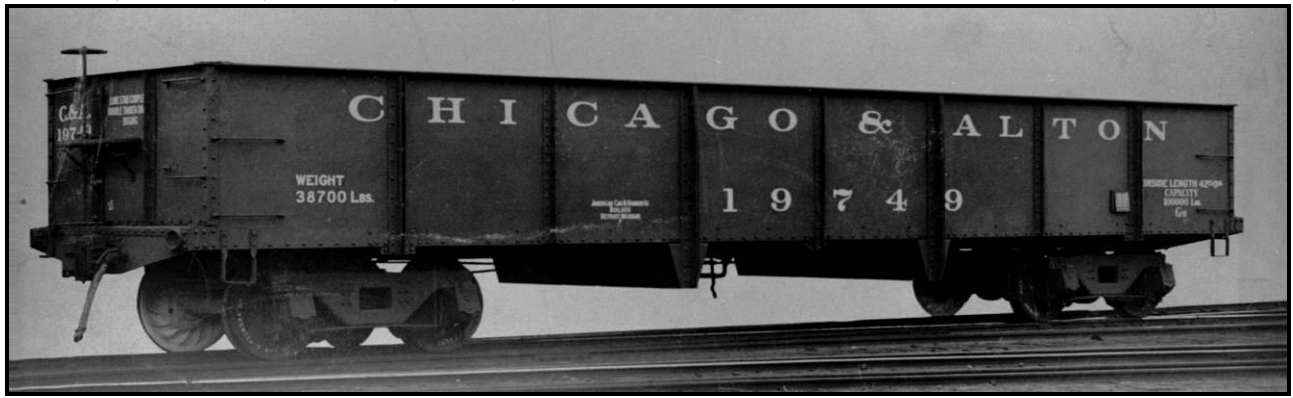
More early all-steel, drop bottom gondolas, there was only one of these cars left in 1927. AC&F builder's photo, Al Westerfield collection.
