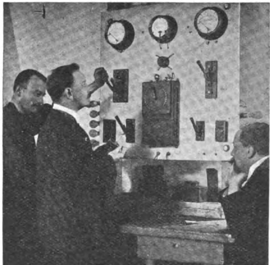
THE DRAUGHTSMAN TESTING A NEW MOTOR FOR CURRENT CONSUMPTION AT THE SPECIAL SWITCHBOARD PROVIDED FOR THIS WORK.
