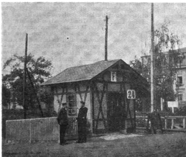
A GERMAN RAILWAY LEVEL CROSSING: VIEW FROM THE ROADWAY.
