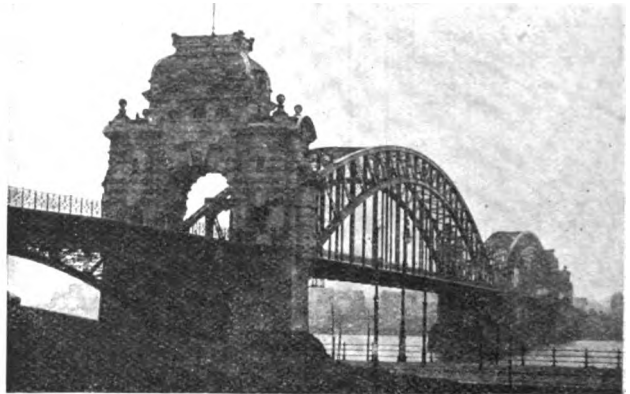
NEW RHINE BRIDGE AT DUSSELDORF, CONSISTING OF TWO ARCHES 197 YARDS WIDE AND 75 FEET ABOVE WATER LEVEL.
