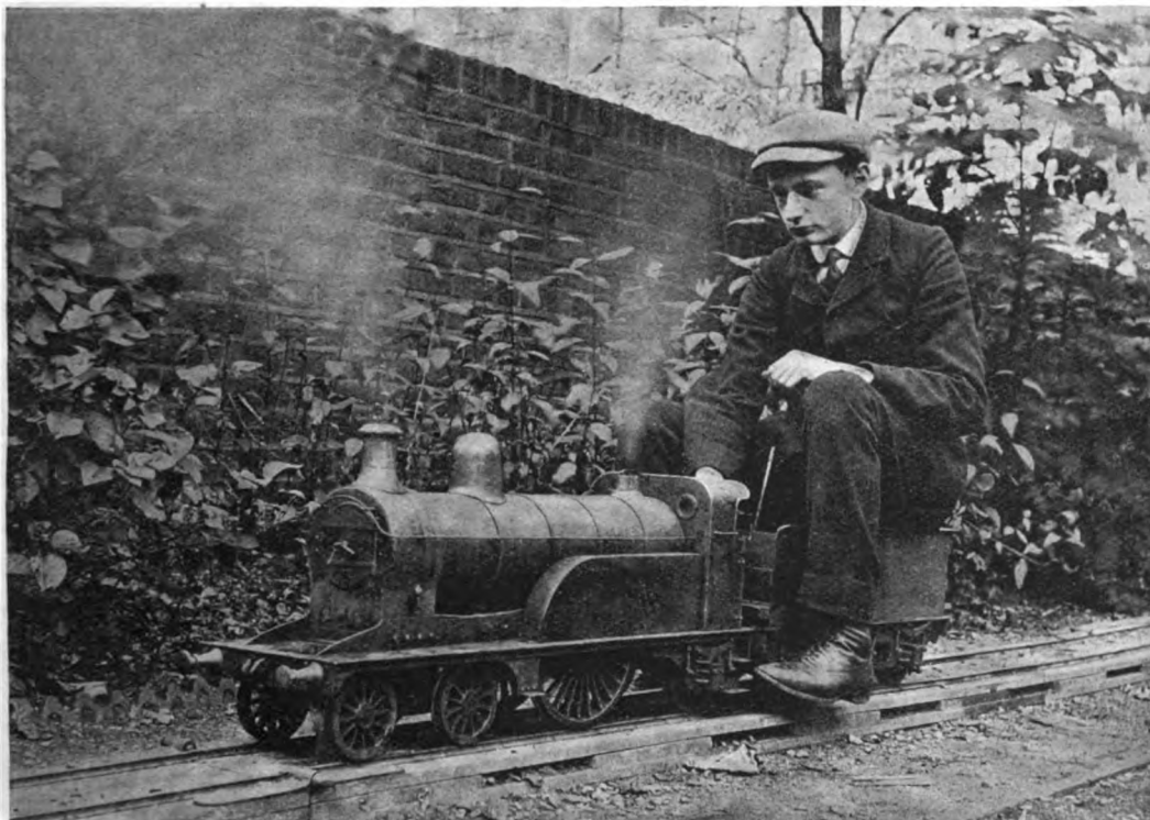
A MODEL 1\frac{1}{4} -IN. SCALE G.N.R. BOGIE SINGLE LOCOMOTIVE.
