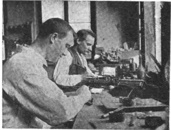
THE PAINTERS AND LINERS AT WORK.
