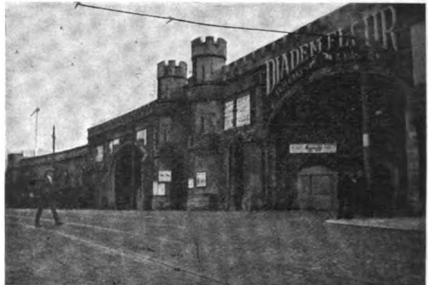
FIG. 19a.—VIEW OF BATH VIADUCT, G.W.R.
