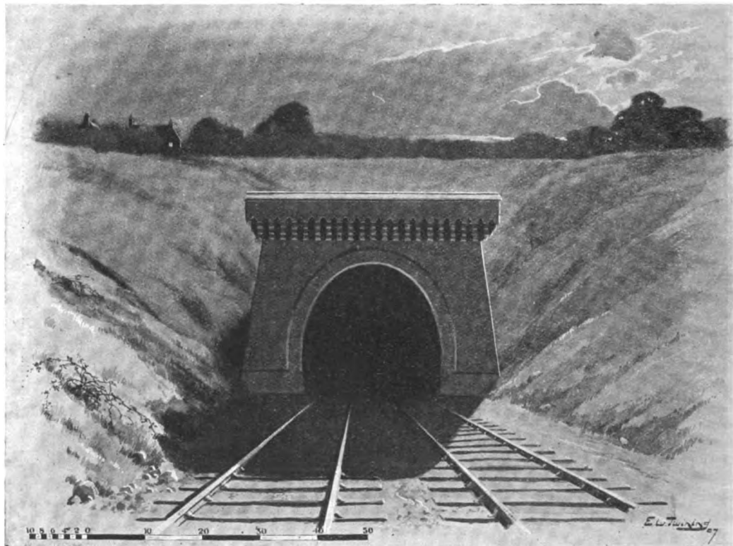
FIG. 15.—NORTHERN END, KILSBY TUNNEL: L.N.W.RY.
