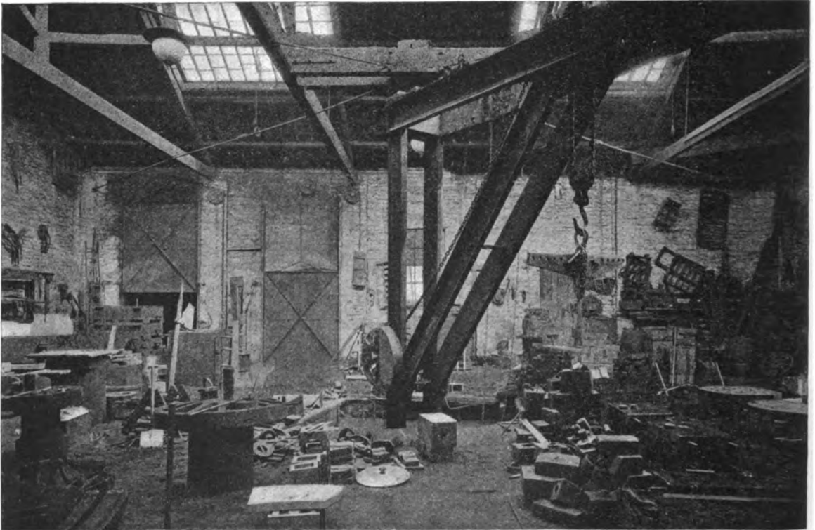
FIG. 9.—VIEW IN IRON FOUNDRY: MESSRS. PECKETT & SONS' WORKS, BRISTOL.
