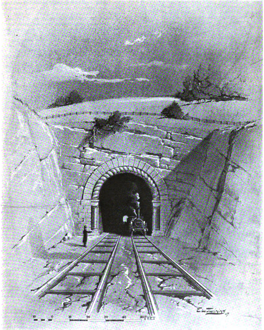
FIG. 1.—WESTERN FACE OF THE ORIGINAL NO. 1 TUNNEL NEAR BRISTOL, G.W.R.
