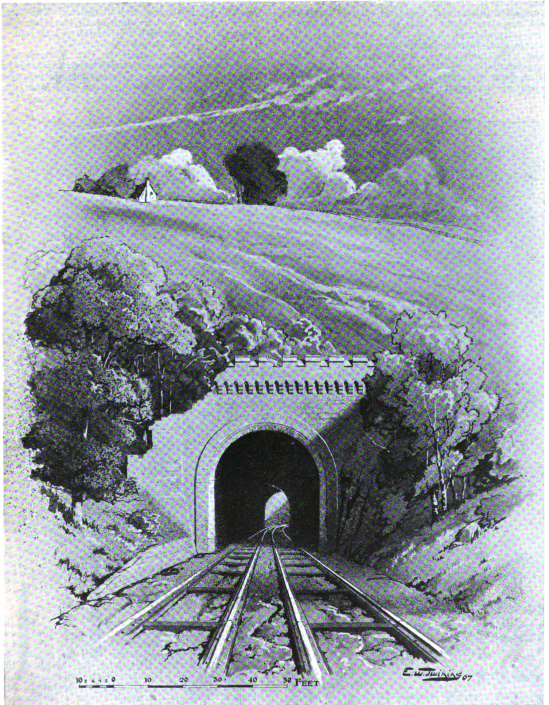
FIG. 2.—WESTERN FRONT OF NO. 2 (NOW NO. 1) TUNNEL NEAR BRISTOL, G.W.R.
