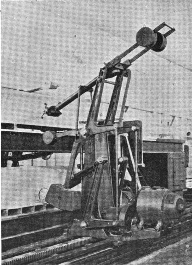
A MACHINE FOR CUTTING MODEL BOAT HULLS.
