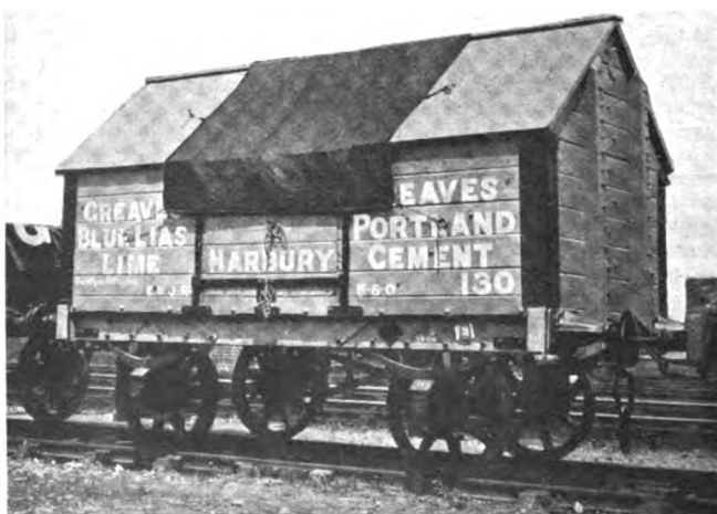
FIG. 16.—PORTLAND CEMENT AND LIME WAGON.
