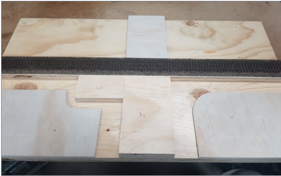
6. The 1/2" plywood cutouts for the roads and railroad service truck easement are in place.
