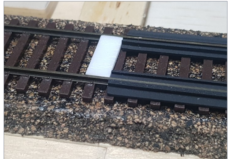
11. Styrene dams for the Smooth-It "Asphalt" are in place.
