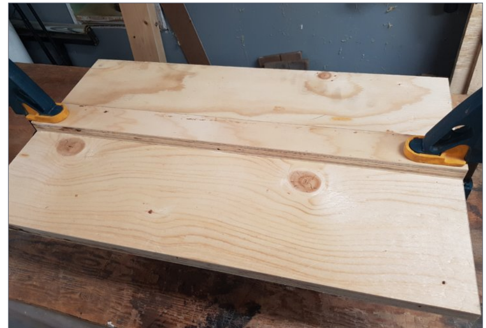
5. The module base with sub-roadbed installed.
