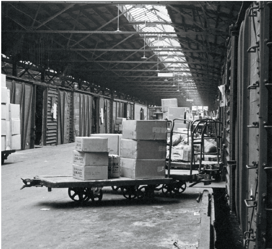
Less-than-carload lot (LCL) package and merchandise traffic lines a covered freight station dock at the Chicago & North Western's Proviso Yard in December 1942. Note the light-colored refrigerator car on the far track. Office of War Information photo, Library of Congress collection
