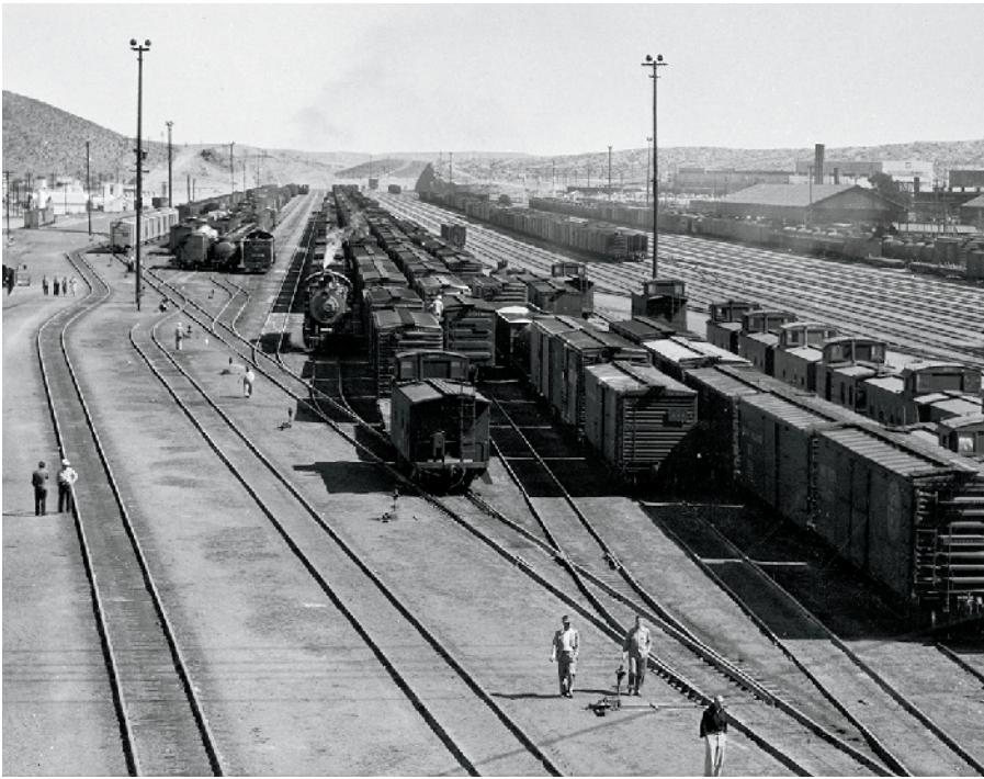
The way car (caboose) tracks at the Atchison, Topeka & Santa Fe's Barstow, Calif., yard were busy in 1948. Train crews ran out of this terminal in three directions – north, east, and west – and every freight train that arrived left with a different way car. Donald N. Nesbit photo
