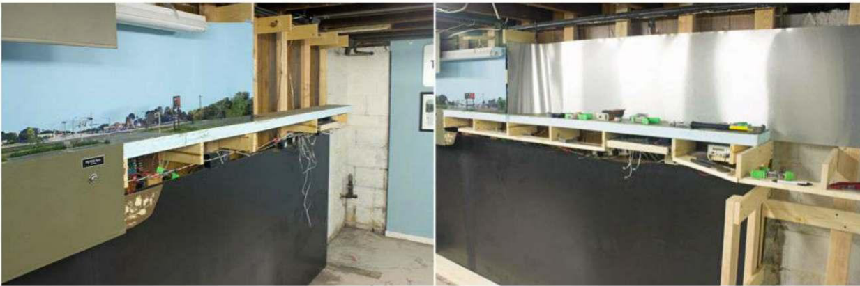
Basic construction methods are evident: 1 x 4 joists overlaid with 2"-thick extruded-foam insulation board. The backdrop is aluminum flashing with photos of the modeled location glued on.
